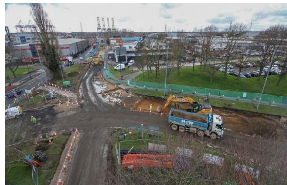
A major programme of road resurfacing and traffic signal upgrades including A33-A35 Millbrook Roundabout.
